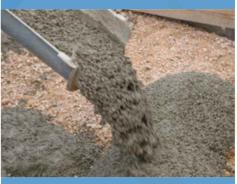
Concrete is also an acceptable sub base. It can be the most expensive depending on your location and square foot area. The concrete thickness should be at least 4" and no less. Be aware that if your area is in a courtyard or difficult to access, you will need a pump truck.
