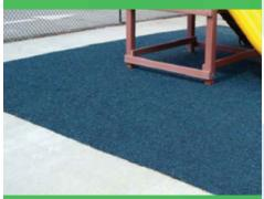
Solid borders are normally formed out of concrete. Keep in mind that when you create a border around your surfacing you are creating a bowl that holds water. There should never be standing water in your surface area. There are many types of drainage options to solve water issues.
