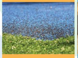
In some cases your new surface may border another type of safety surface. In the picture above this is EPDM against artificial turf. Depending on the two types of surface and the fall height, the mechanics to connect the two can vary.
