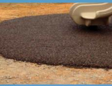
The rolled edge application is the most commonly used method. The edge of the surfacing will die into a trench around the sub base. After the surfacing is installed the dirt from the trench is used to backfill against the surfacing.
